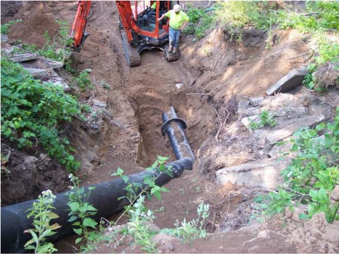
Emergency Repair of washed out culvert
