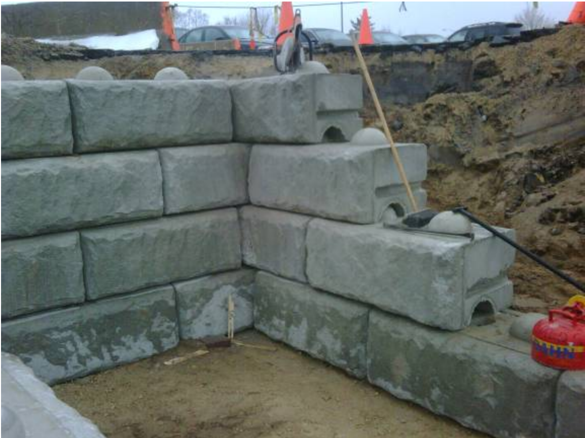
Detail of wall corner installed by Dahn Construction crews.
