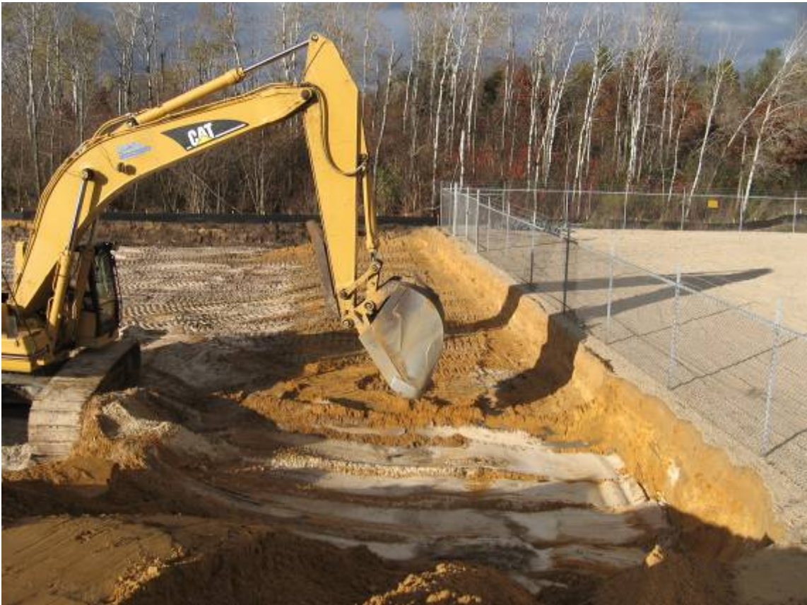
Grading for expansion of an existing substation in Western Wisconsin
