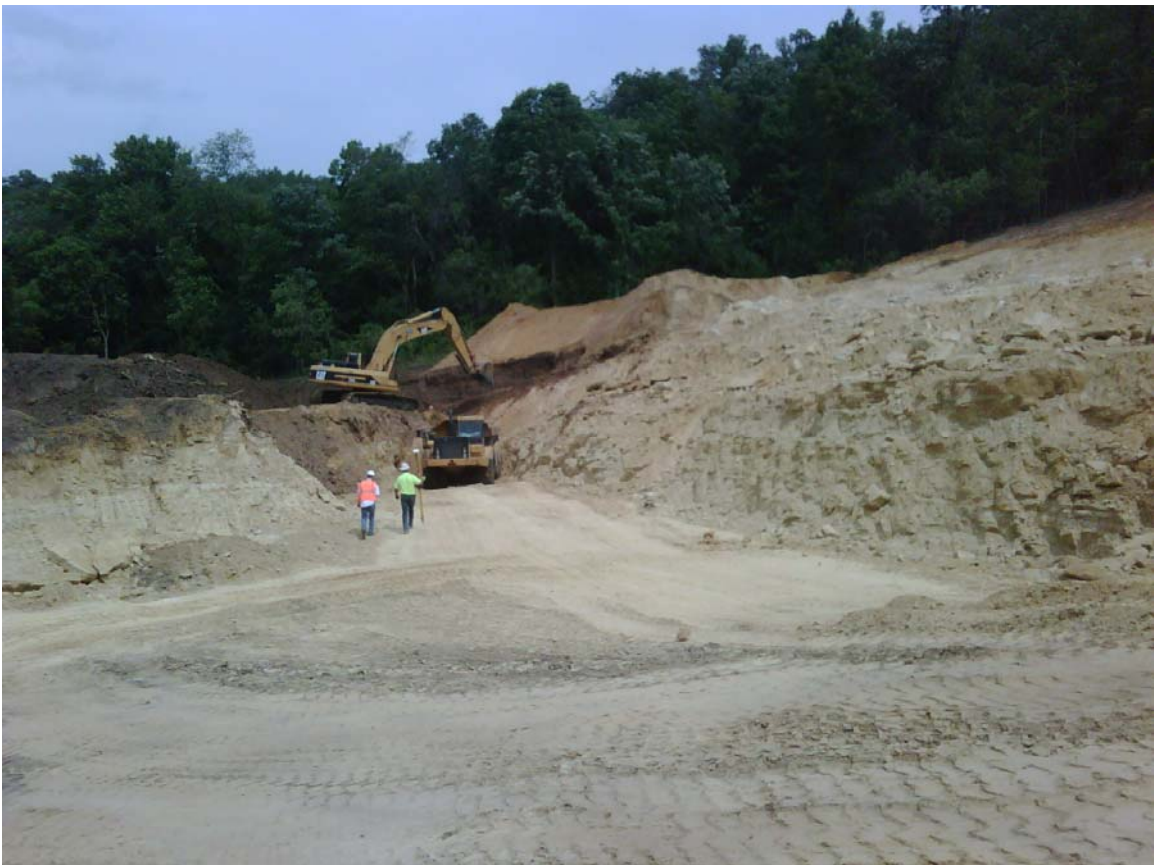
Borrow Excavation for construction of a new landfill cell.
