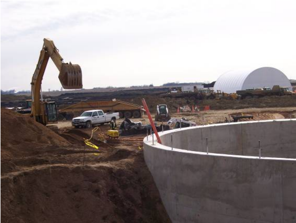
Grading around tanks at Welcome Ethanol Site
