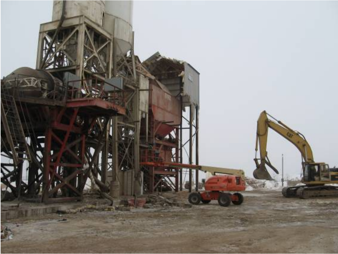
Demolition of a batch plant in Dayton
