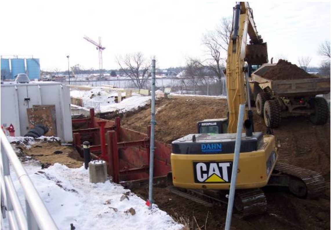
Installation of 96" FRPMP pipe at Blue Lake WWTP
