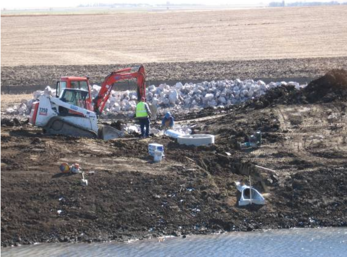
Pipe, structure, and riprap installation for sub station grading project
