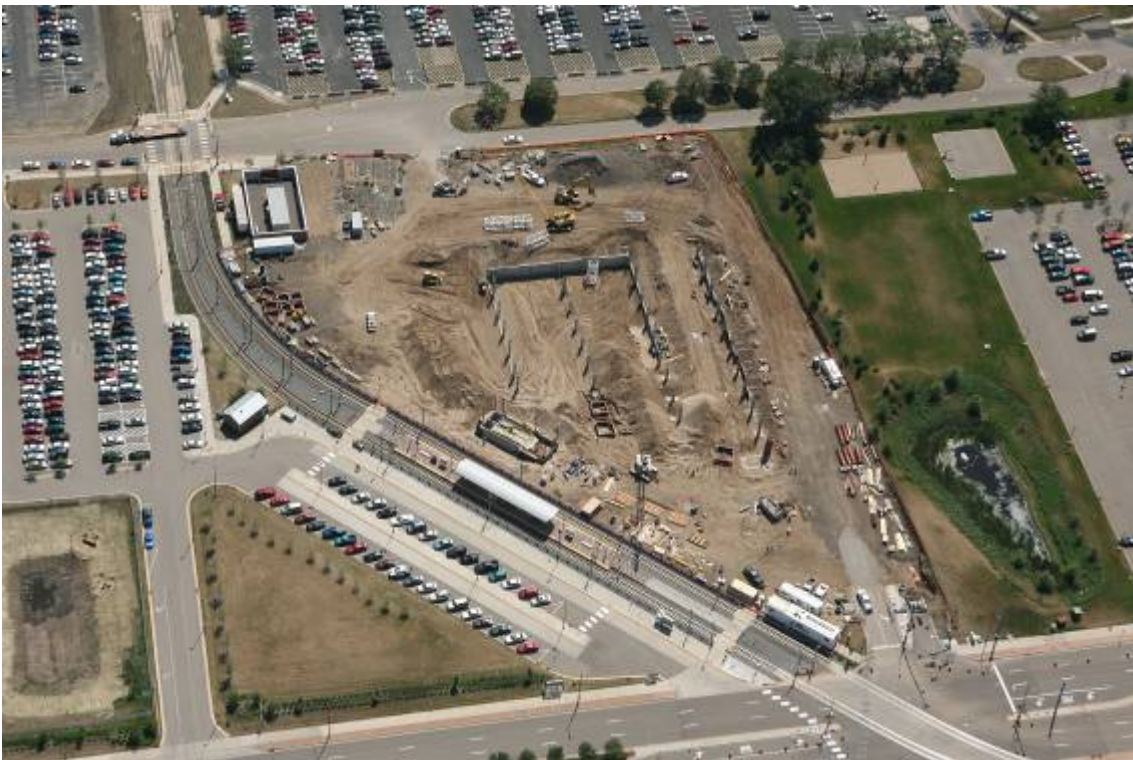
Aerial photo of grading project for LRT Parking Ramp in Bloomington
