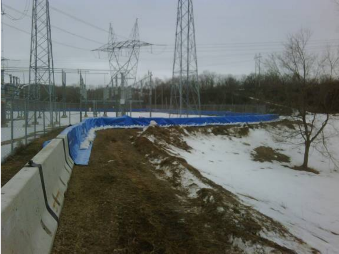
Flood Wall under Construction using barriers and polywrap.
