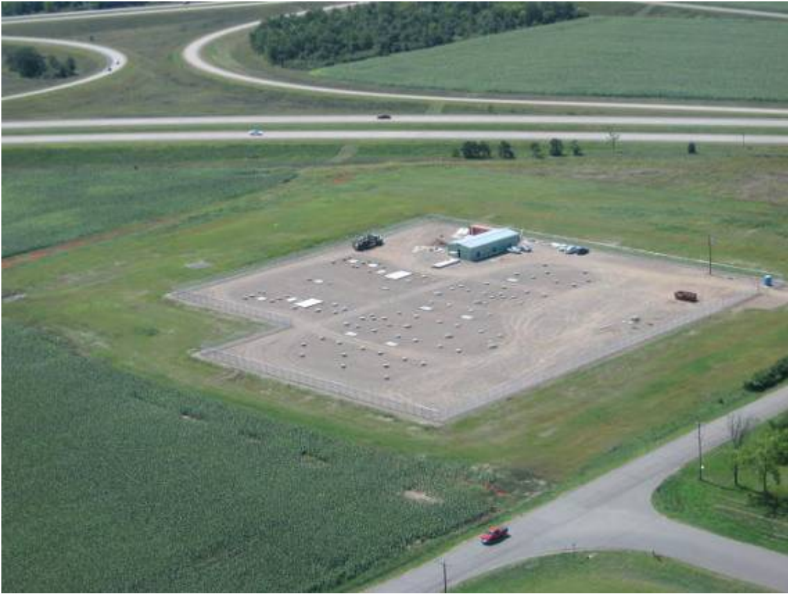
Aerial view of a completed substation in Central Wisconsin
