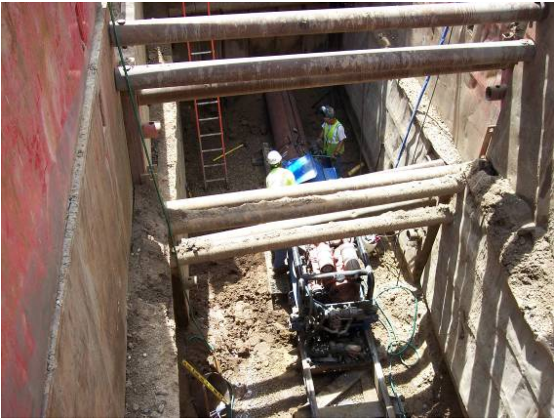
Jack and Bore for Sewer line under UPRR
