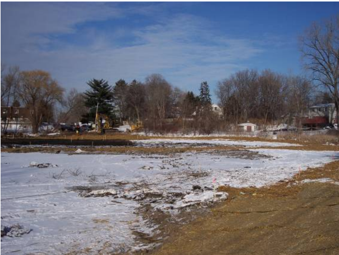
Finish grading and restoration at South St. Paul Pond Project
