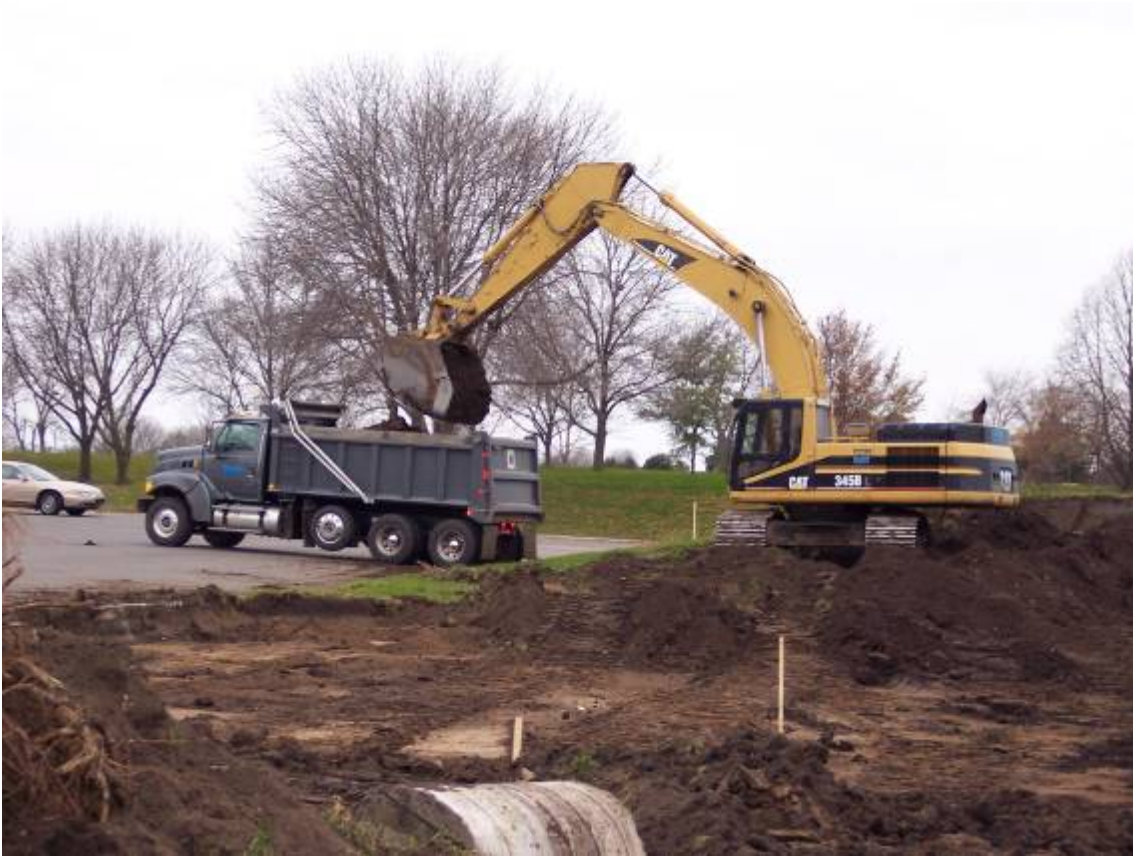
Grading for new parking lots at Dakota County Technical College
