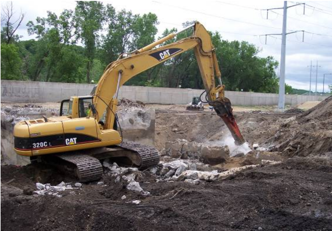
Demolition of old substation and footings in St. Paul
