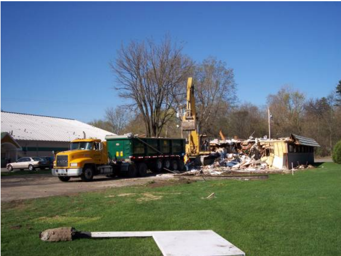
Demolition of Commercial Building in Minnetonka
