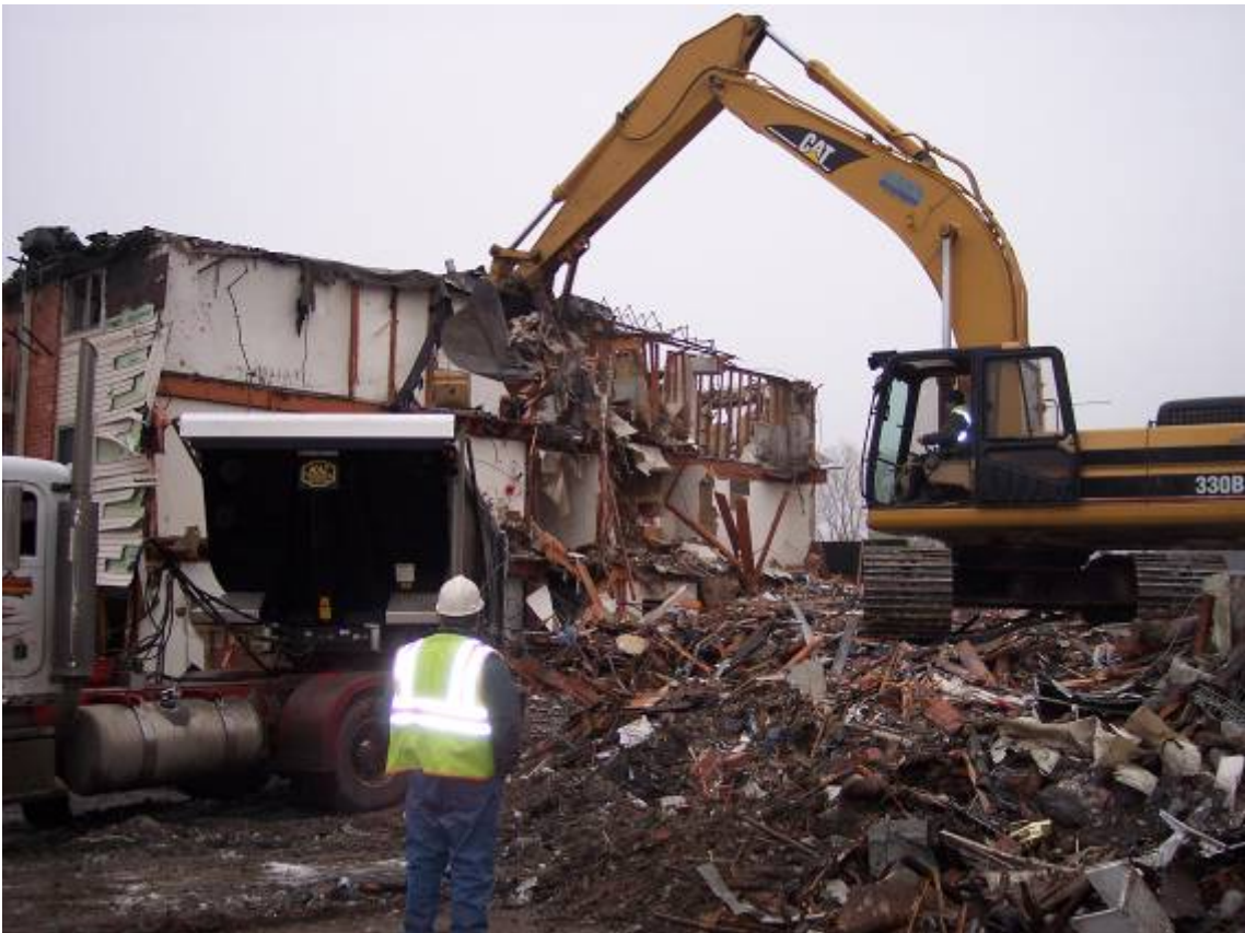
Demolition of Burncliff Apartments in Burnsville
