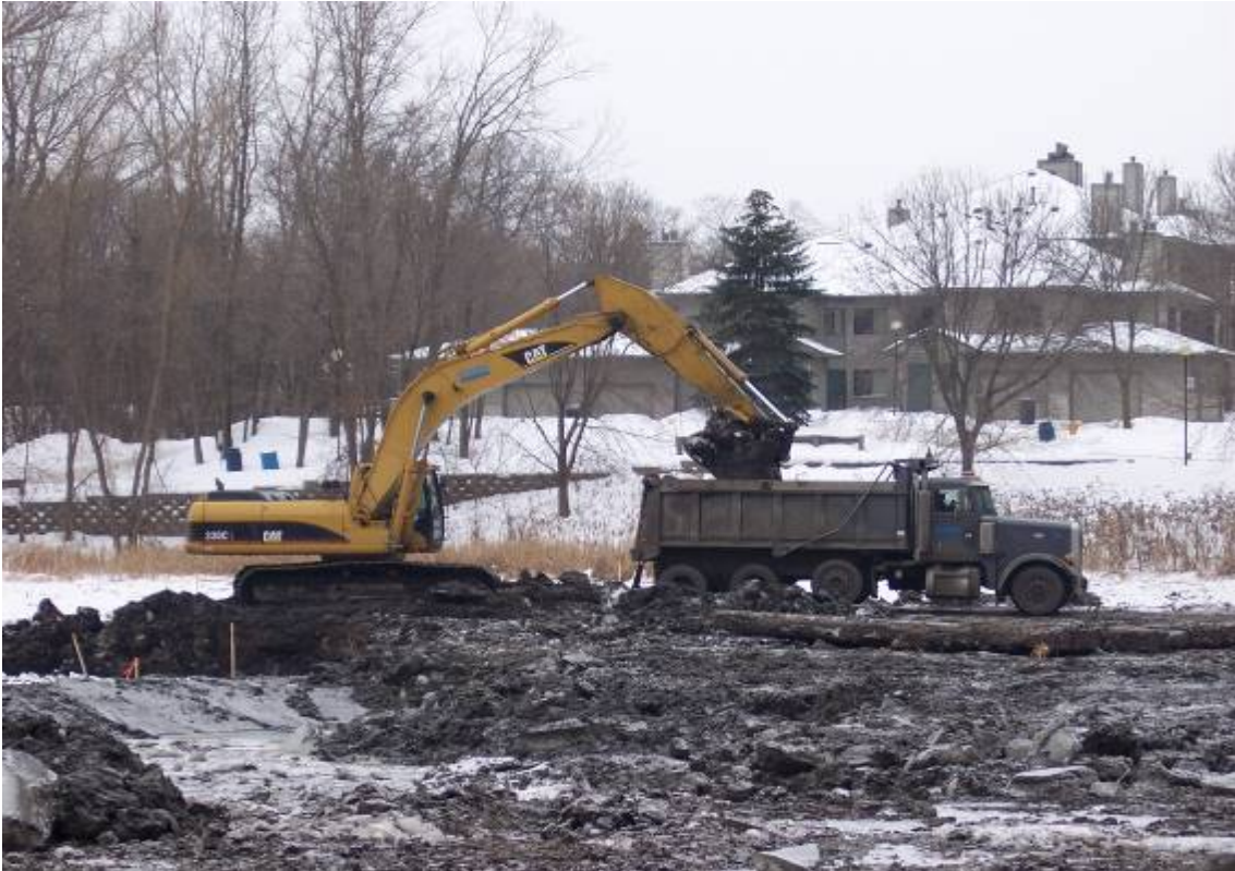
Exporting and grading to enlarge an existing pond in South St. Paul
