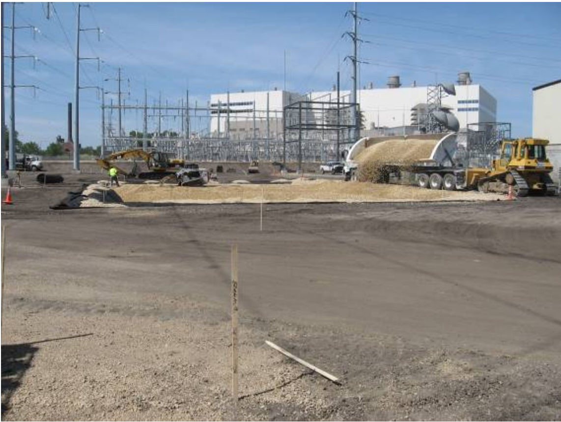
Grading for infiltration area at live substation
